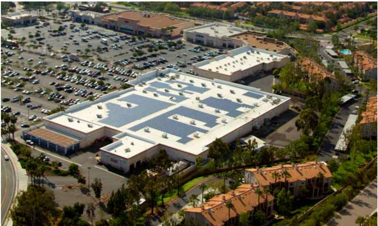
A Walmart location uses solar panels to generate power in Corona, CA.
