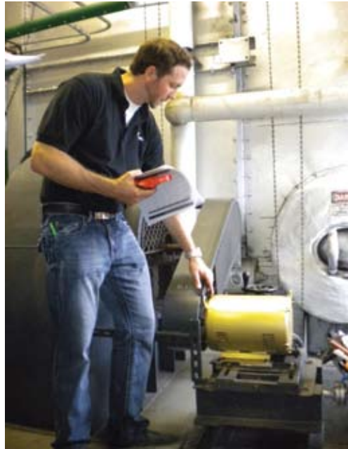
Energy audits have helped identify opportunities for improving energy efficiency. Credit: NREL.
