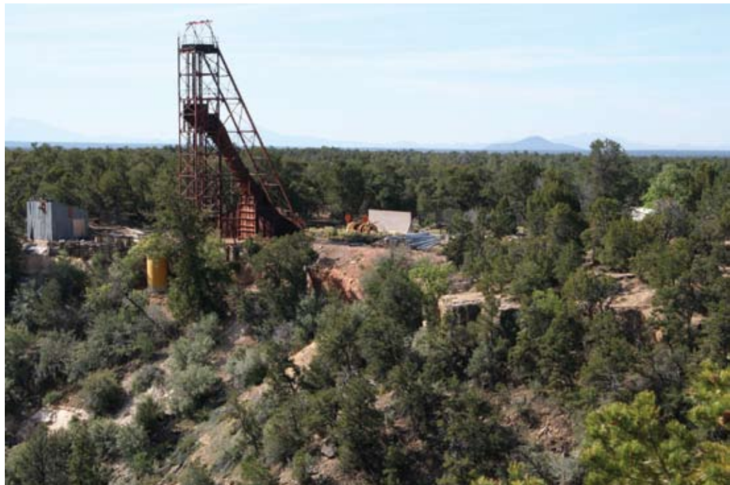
Abandoned equipment and structures for the Orphan Mine on the rim of the Grand Canyon in 2007, decades after the mine closed and shortly before the National Park Service removed them from the site. Photo: Alan Levine via Flickr, public domain.
