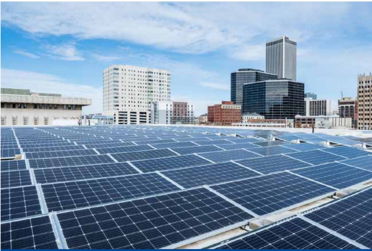
Solar panels overlook the Tulsa skyline from the city's Central Library.
