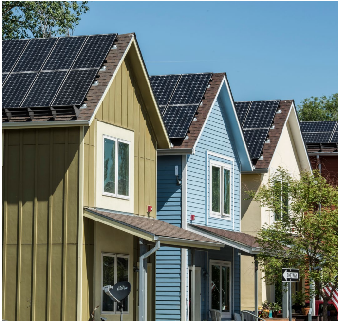
Solar panels atop homes in Boulder, CO
