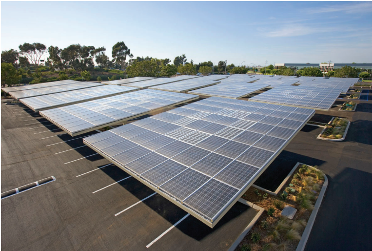
With “vehicle to home” technology, plug-in car owners could charge their cars during the day at solar parking lots—such as this one at Kyocera’s employee parking lot in San Diego, California—then use remaining battery power after they drive home to help power their houses in the evening. Photo credit: Envision Solar.
