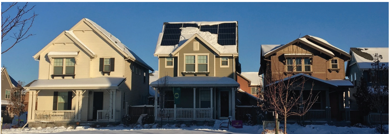
Solar panels on a home in Denver, CO.
