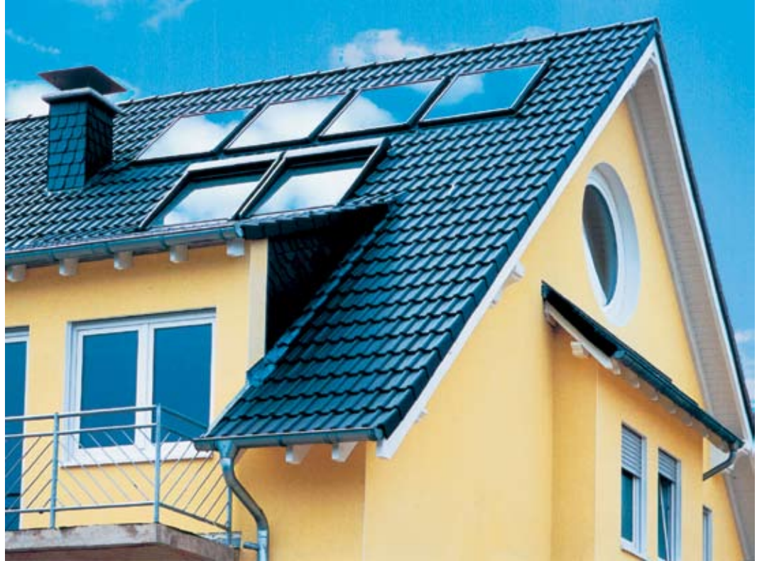
Solar water heating systems, which are common in parts of the world, can provide 50 to 80 percent of a building's hot water needs. Credit: VELUX/ESTIF
