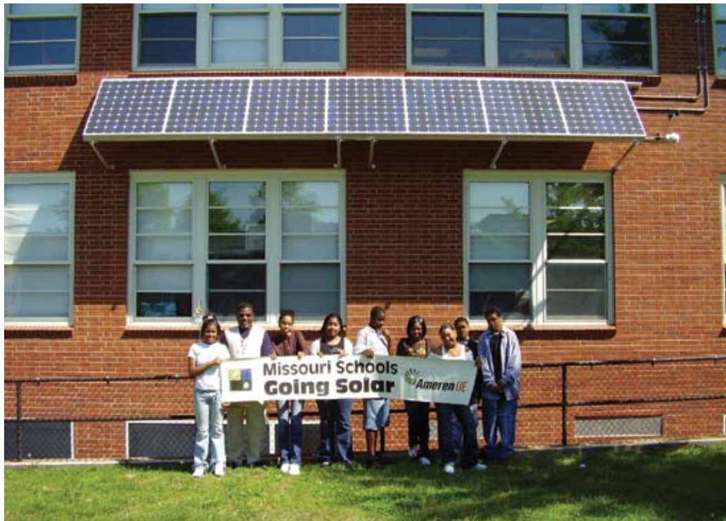
Government can help spur the development of a solar economy by taking the lead in installing solar energy systems on public buildings, such as this middle school in Missouri. Credit: Missouri Department of Natural Resources
