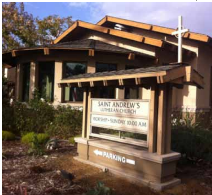
St. Andrew's Lutheran Church in Mar Vista installed its panels in October 2013.
