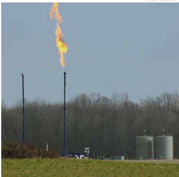
Flaring in Scott Township, Lawrence County, Pennsylvania.
