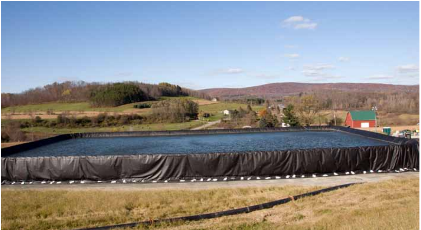
A fluid retaining basin at a Marcellus Shale site in Pennsylvania.
